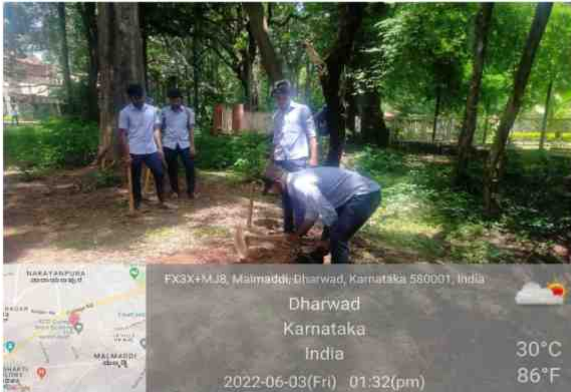
Digging pits and cleaning the campus.
